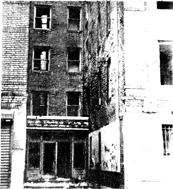
Abandoned Building — 634 Fox Street Bronx. Domingo Acevedo and Jeromino Pena are registered to vote under this address.
